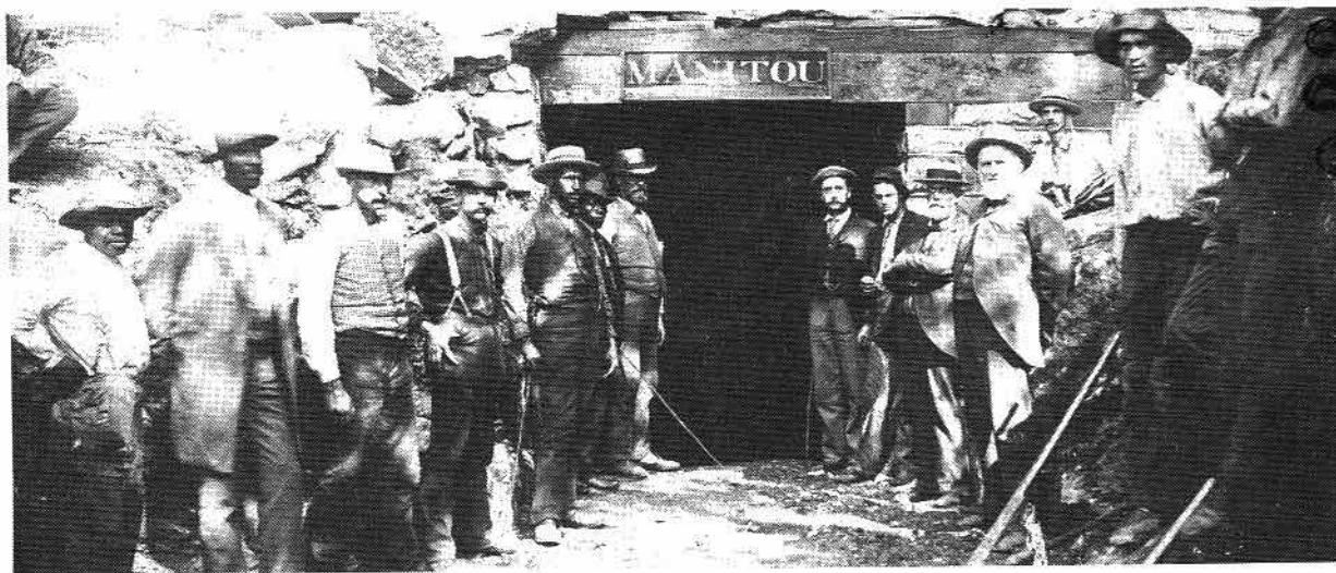
A group of local citizens photographed at entrance to MANITOU Cave in south Fort Payne about 1878. Those identified are Harry Reed Godfrey and Orlando Godfrey, second and third on right, respectively, and Captain William H. H. Minot, on left of cave entrance in straw hat. In cave entrance, left, Archie Spaulding; right, Mort Spaulding.
